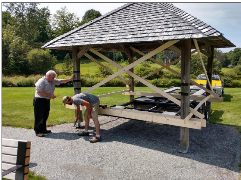
GLEN AND CODY FINE-TUNE THE INSTALLATION
